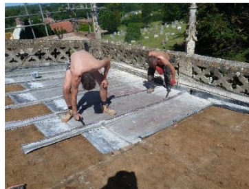
Stripping the remaining lead...
