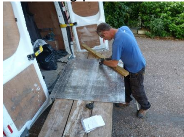
Marking up the lead sheet
