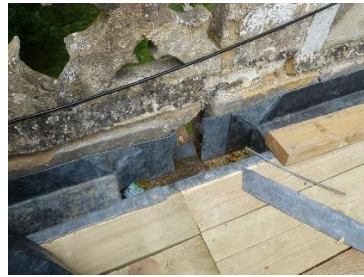
Gutter sump in position
