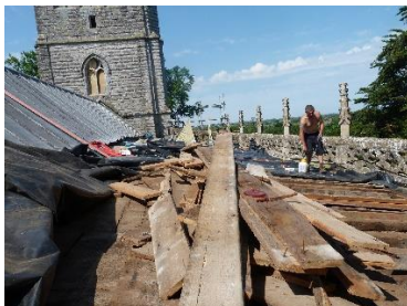
Timbers are lifted...
