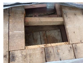
Discovery of the steel girder
