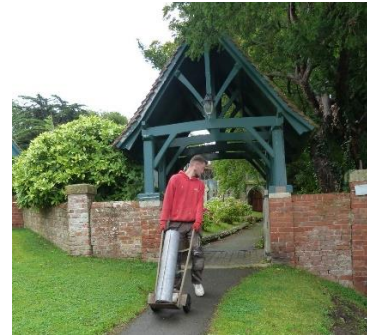
..and wheeled to the scaffolding
