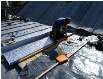
Placing the mopstick
