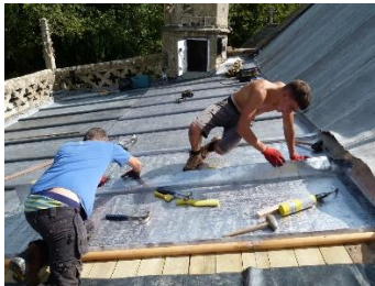
Rolling the lead over the mopstick
