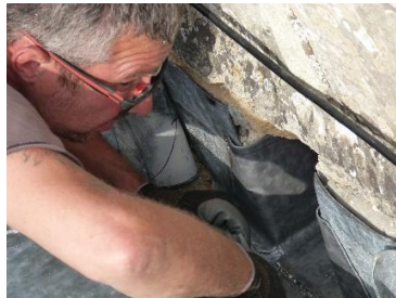
Sump/spout welds being cleaned
