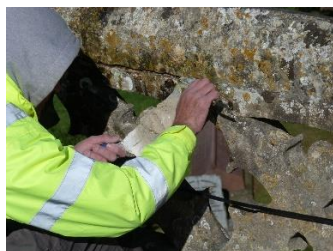
Repointing with lime mortar
