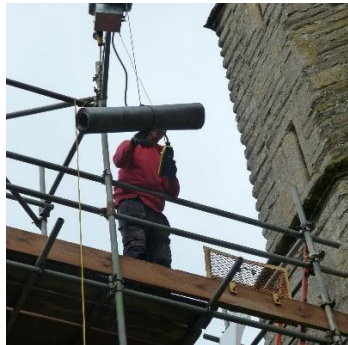
Winching 100kg of lead appears to be quite easy...
