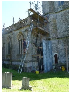
Scaffolding is erected
