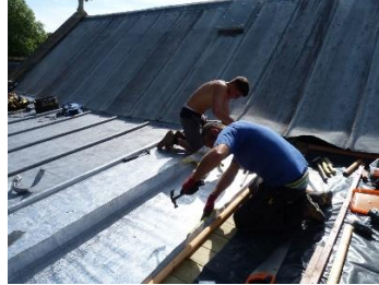
Hammering the lead into position
