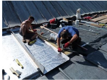
Fixing the mopstick in place
