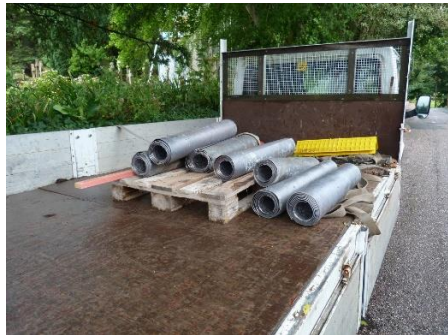
Lead rolls arrive on site in 100kg rolls
