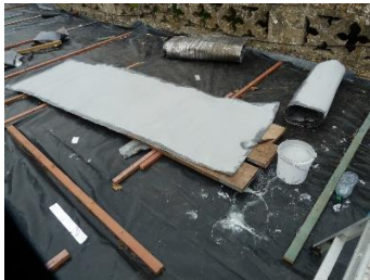
Lead roll with painted underside
