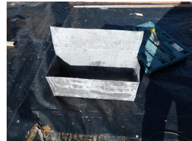
A finished product – a gutter sump
