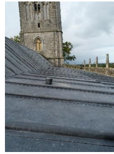
The finished roof
