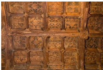
Panels of the ceiling
