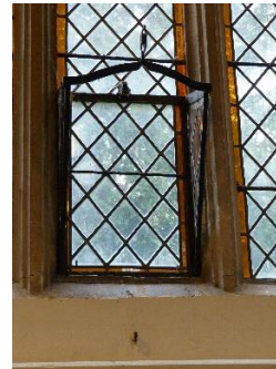
Window iron work
