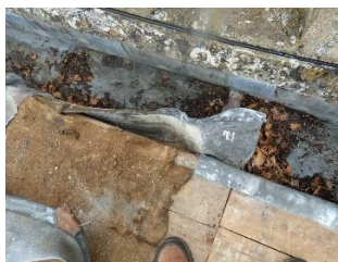
Lead gutter on a concrete base
