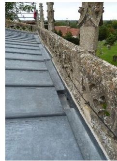
Finished gutter
