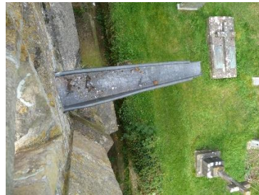
Water spout in position
