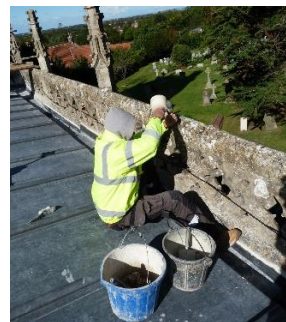
Raking out old mortar
