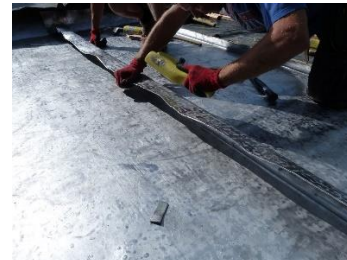
Hammering the lead down
