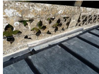
Chasing in the lead flashing
