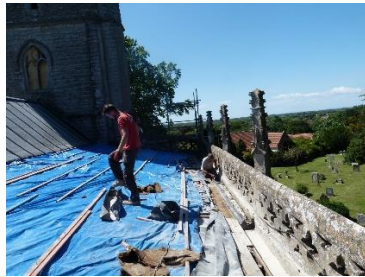
Overlength gutter being removed
