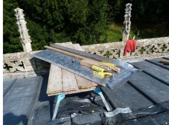
Constructed "bay box"
