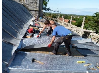
Putting a bay box in place
