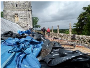
Rolling back the covers for inspection
