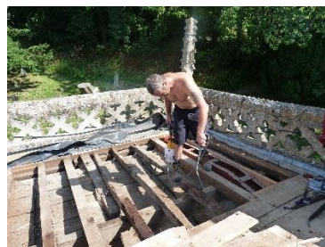
and underlying wood is treated
